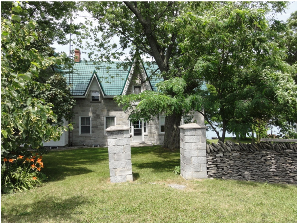
Plate 8: 3190 Front Road, Gothic Revival Cottage wing
